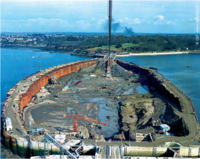
The power station under construction
